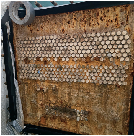
End cap removed and exchanger tubes are sealed with corks prior to surface prep.
