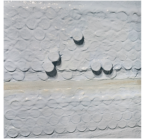
Metal loss is rebuilt, then first step of Belzona 1341 gray coating is applied.
