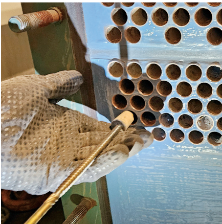
All sunken corks are removed from within the heat exchanger tubes.
