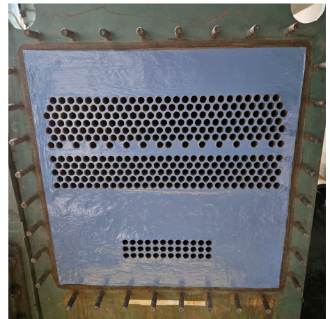
Completed tube sheet restoration ready for service after final inspection.
