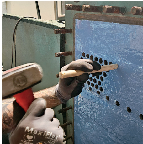
Corks are tapped into exchanger tubes after coating has cured.
