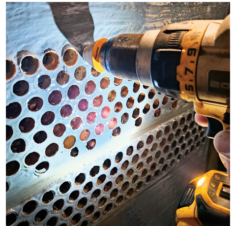
Tube ends are chamfered to remove residual coating overlap.
