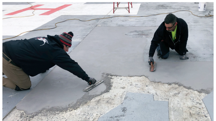
Areas of concrete damage cut out and patched with Belzona 4131.
