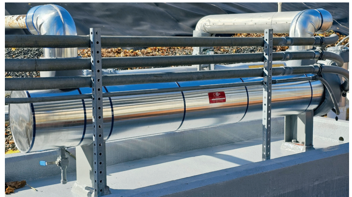
Cylinders were re-insulated after repair and coating application.
