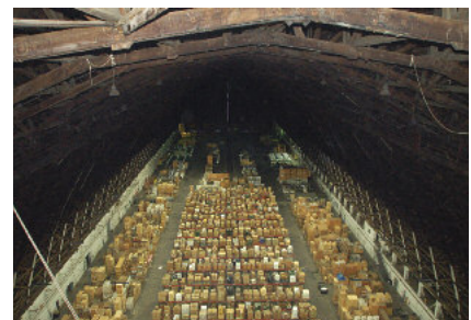
View of warehouse area from the ceiling.
