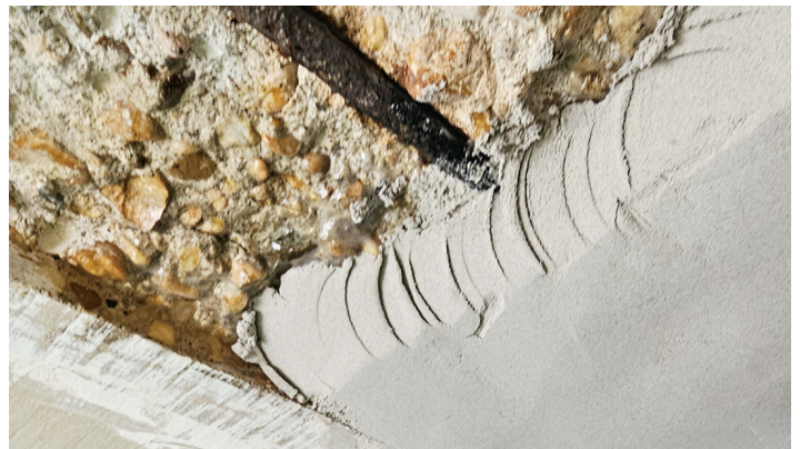
Belzona 4141 is applied overhead without formwork.
