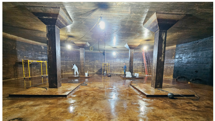
Surface prep of 10,000 sq. ft. underground water storage tank.
